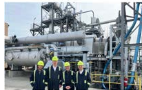
Alterra chemical recycling plant, Akron, OH
